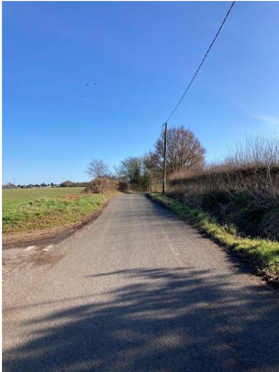
39. Junction of Kelvedon Road and New Road. No signs in New Road. Road is bordered by deep ditches
