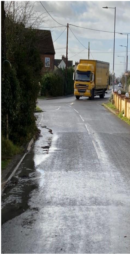
58. Accident black spot for obscured right turn
