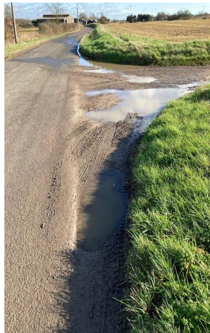
6. Extensive damage and destruction to road edge
