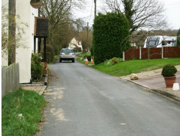
45. Showing the road width from 120m onwards
