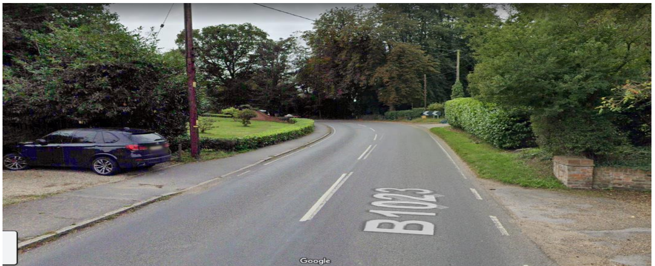
B1023 approaching All Saints Church (looking south) – shows frequency of accesses, narrow verges, low radius (approximately 75m) curve and limited visibility.
