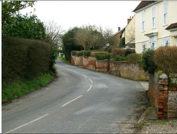
20. Looking up Harborough Hall Lane showing the brick wall outside the Bell House
