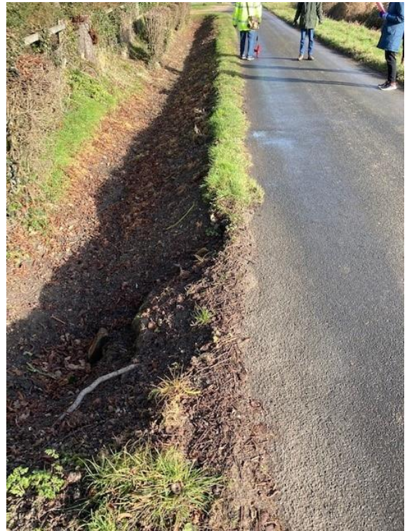
47. To show deep ditches within 20cm of road edge. No signs, no warning
